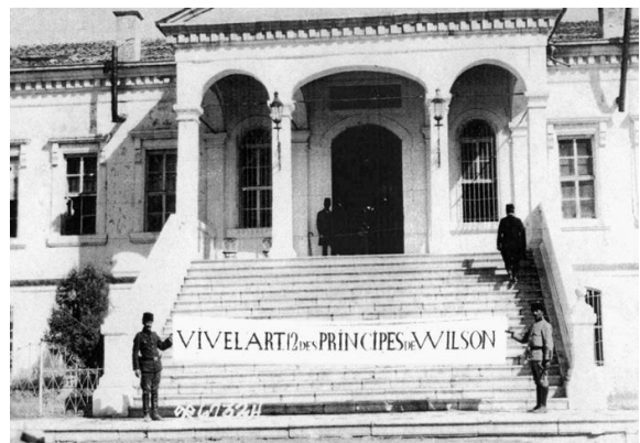
Figure 8.2 The Courthouse at Erzincan, September 24, 1919.
